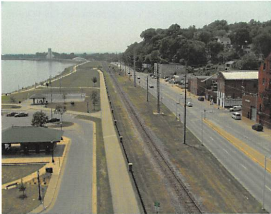
Mississippi Drive Corridor
