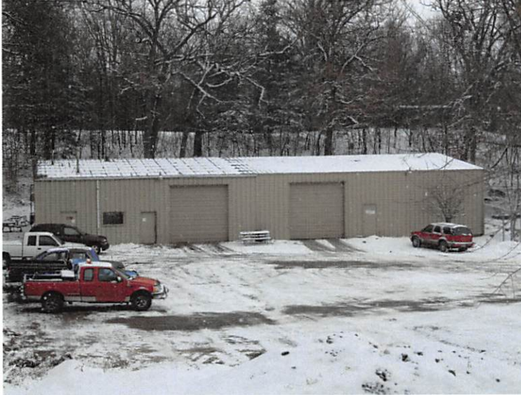
Weed Park Maintenance Shop
