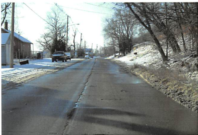
Hershey Street Reconstruction
