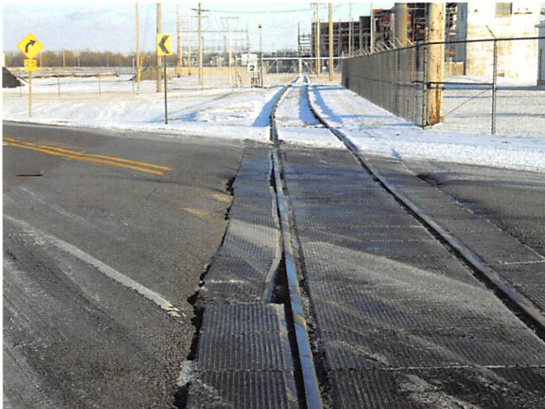
Railroad Crossing on Dick Drake Way at MP&W Gate #2
