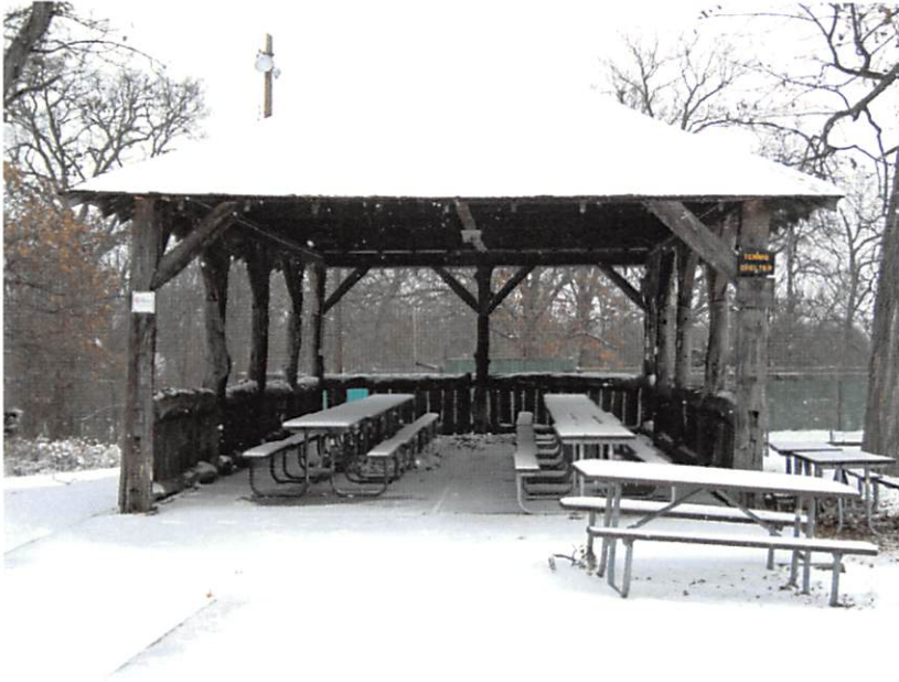
Weed Park Shelter
