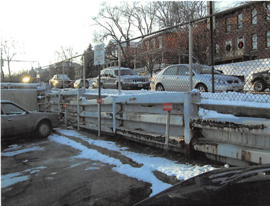
Third Street Parking Lot Retaining Wall
